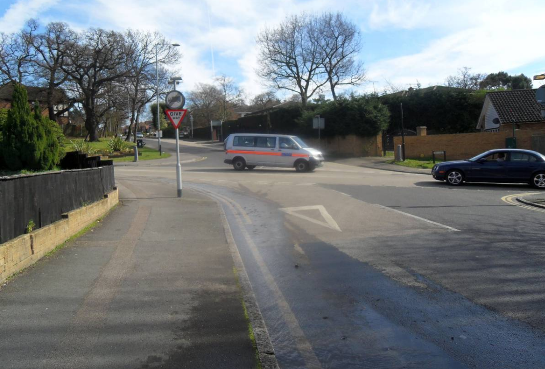
Photograph 8. On Turpins Lane, approaching the junction
