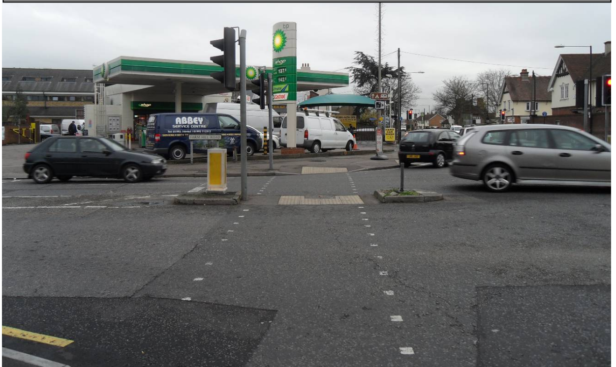
Photograph 3. Pedestrian crossing at Farm Hill Rd signals east of junction
