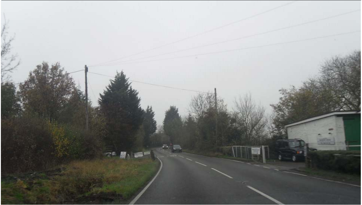
Photograph 1. Northbound, approaching the right hand bend
