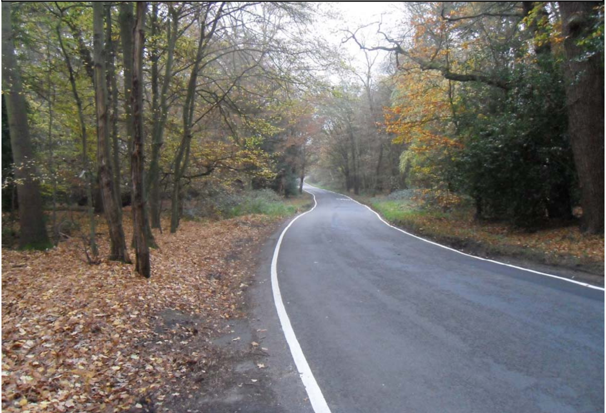
Photograph 1. Claypit Hill northbound
